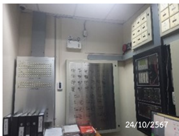
Graphic Annunciator Fire Alarm System
