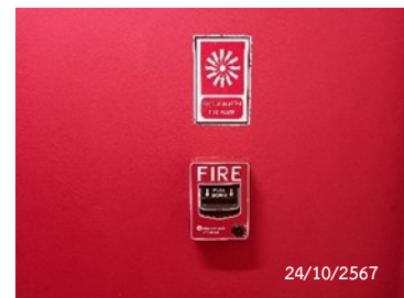
Fire Alarm Manual Station
